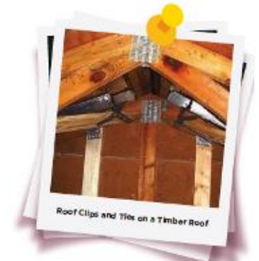
HURRICANE/WIND ROOF ANCHORAGE
